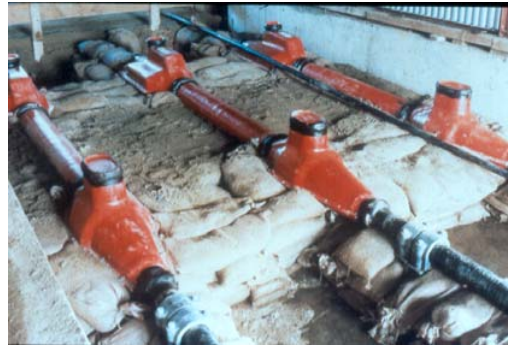
A buried joint bay during the backfill operation
