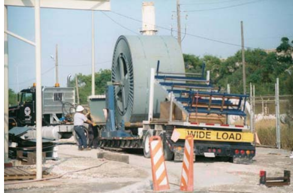
Reel being prepared for cable pulling
