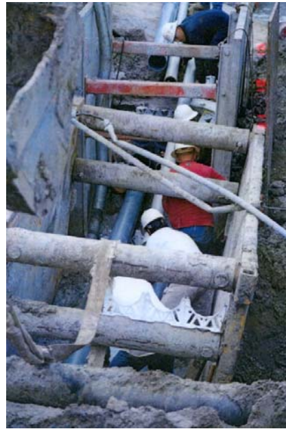
Ducts being positioned in a deep trench before pouring concrete
