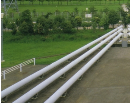
GIL installed on short stilts (diagrammatic representation only)
