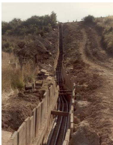
Open cable trench
