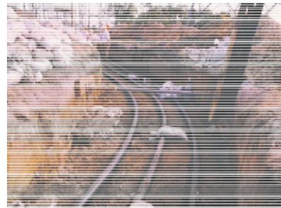
Three parallel lines or cables are required to form a circuit
