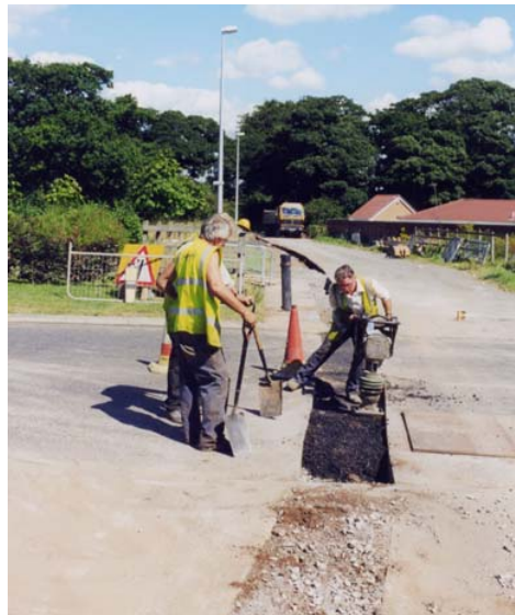
Temporary trench reinstatement
