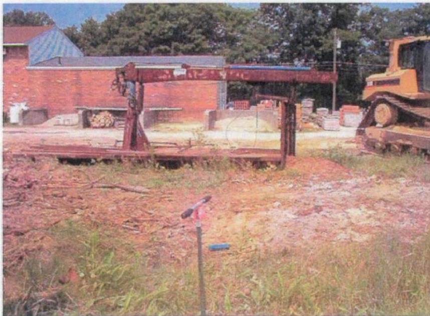
Rear of landscape business located at 347 Riverside Drive. View looking west
