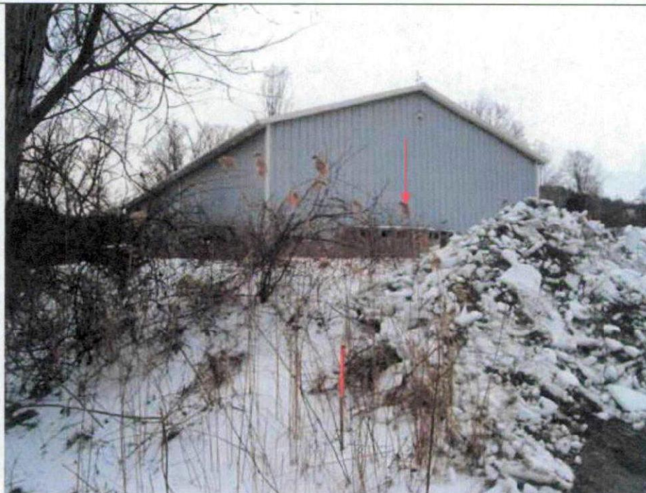
6. View of the proposed tower site from the northwest.
