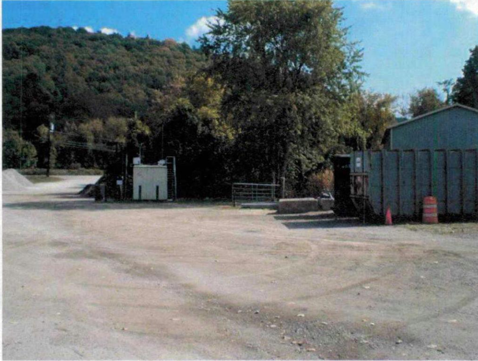
Photo 1 : View of transfer station gravel drive with Wetland 1 in background and proposed Verizon Wireless facility to the right near dumpster and just out of the photo, looking northeast.
