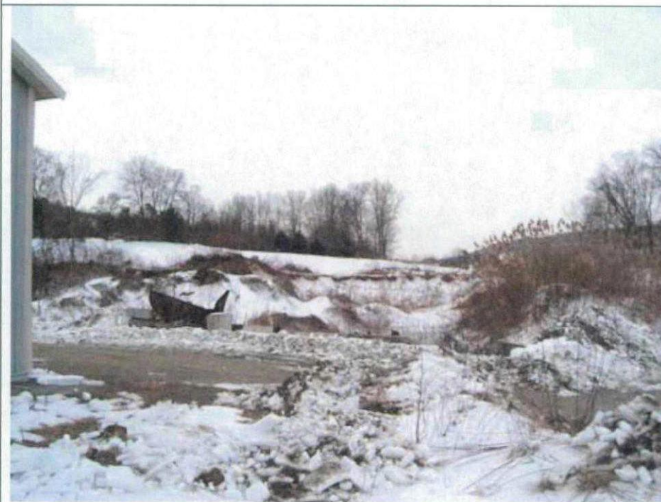
4. Facing south from the proposed tower site.
