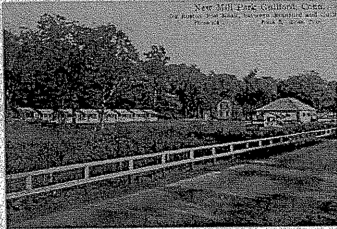
EARLY PHOTOGRAPH OF THE NEW MILL PARK CABINE ON BOSTON POST ROAD WEST
