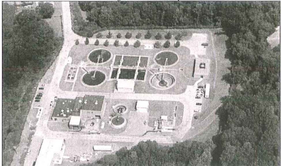
Sewage Treatment Facility
