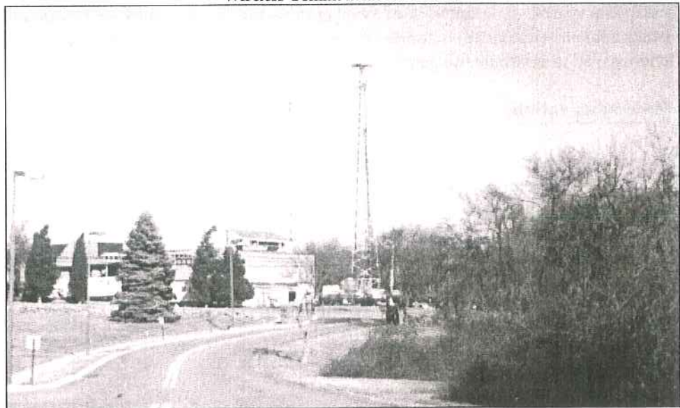
Wireless Communication Towers
