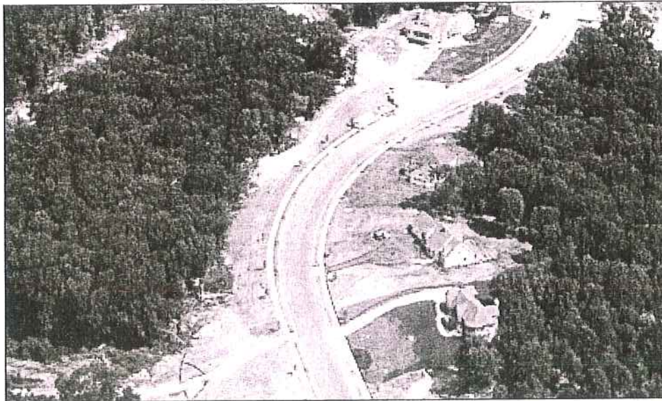
New Road and Sidewalk Construction
