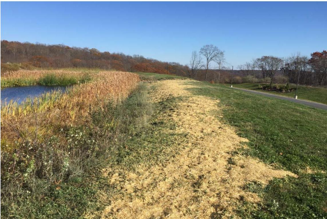
Photo 25: View of Basin 'A' side slope areas hydroseeded and mulched looking east.
