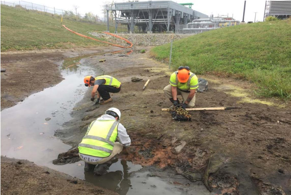
Photo 19: View of Basin 'B' high marsh replanting work looking south with micropool in background.
