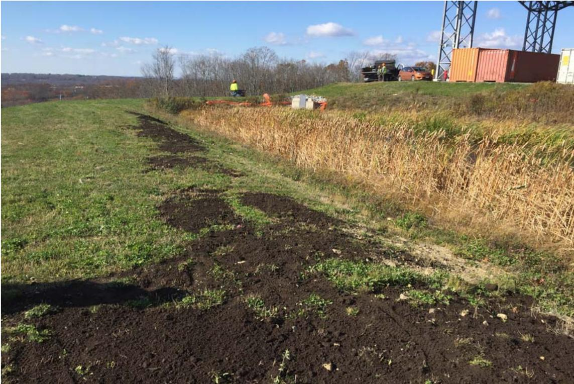
Photo 24: View of Basin 'A' side slope areas stabilized with loam looking west.
