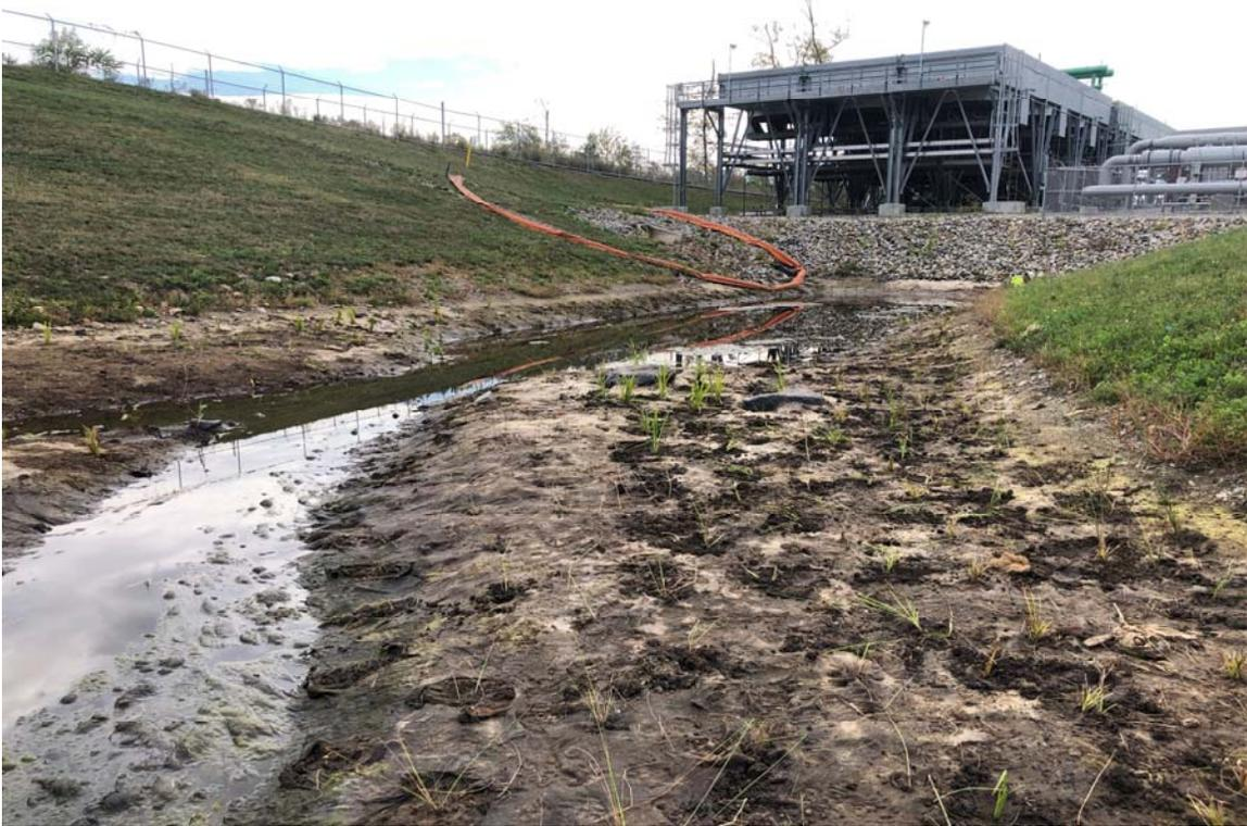
Photo 21: View of Basin 'B' completed replanting of high and low marshes looking south with micropool in background.
