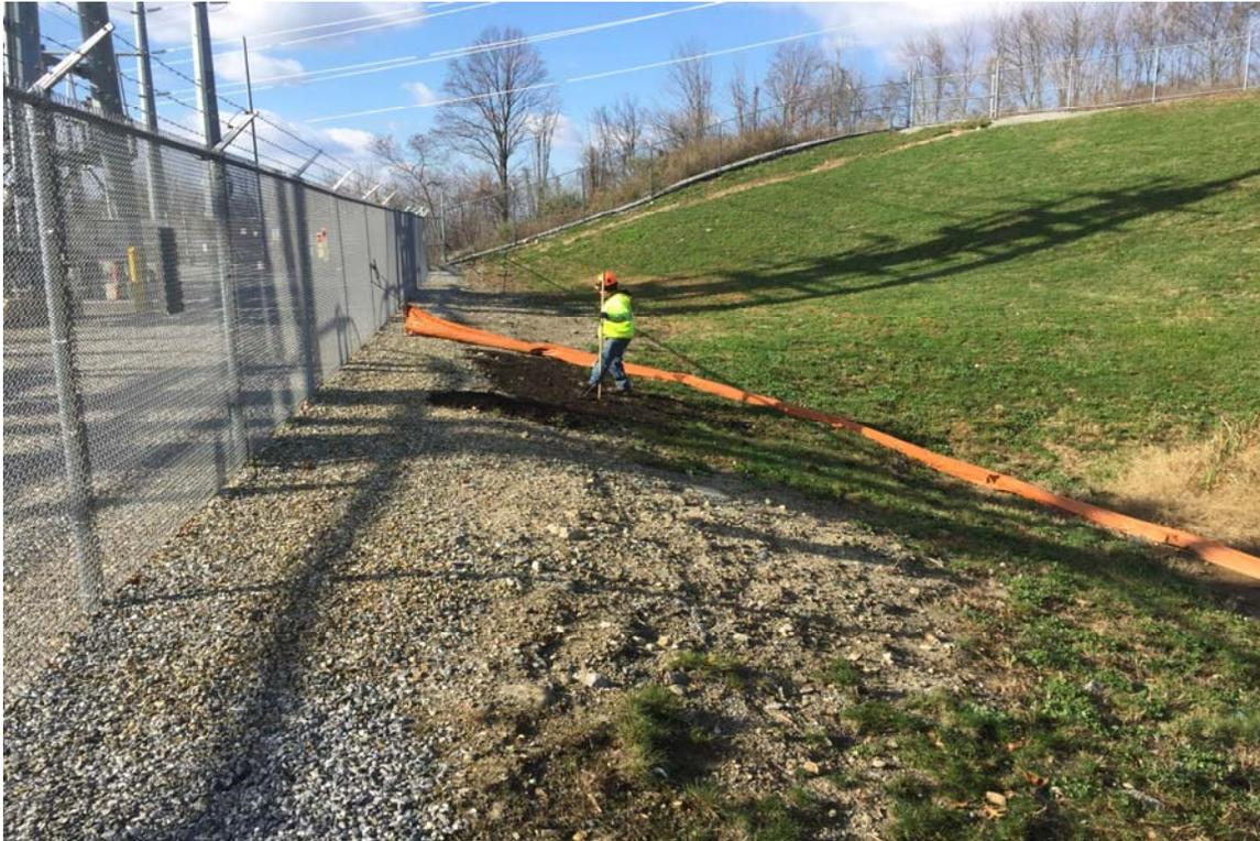
Photo 22: View of Basin 'B' side slope areas being stabilized with loam looking west.
