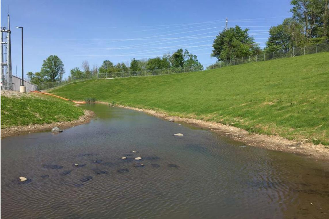
Photo 13: View of Basin 'B' high and low marshes (general lack of vegetation) looking west with forebay in background.
