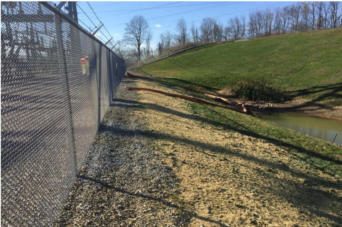
Photo 23: View of Basin 'B' side slope areas hydroseeded and mulched looking west.
