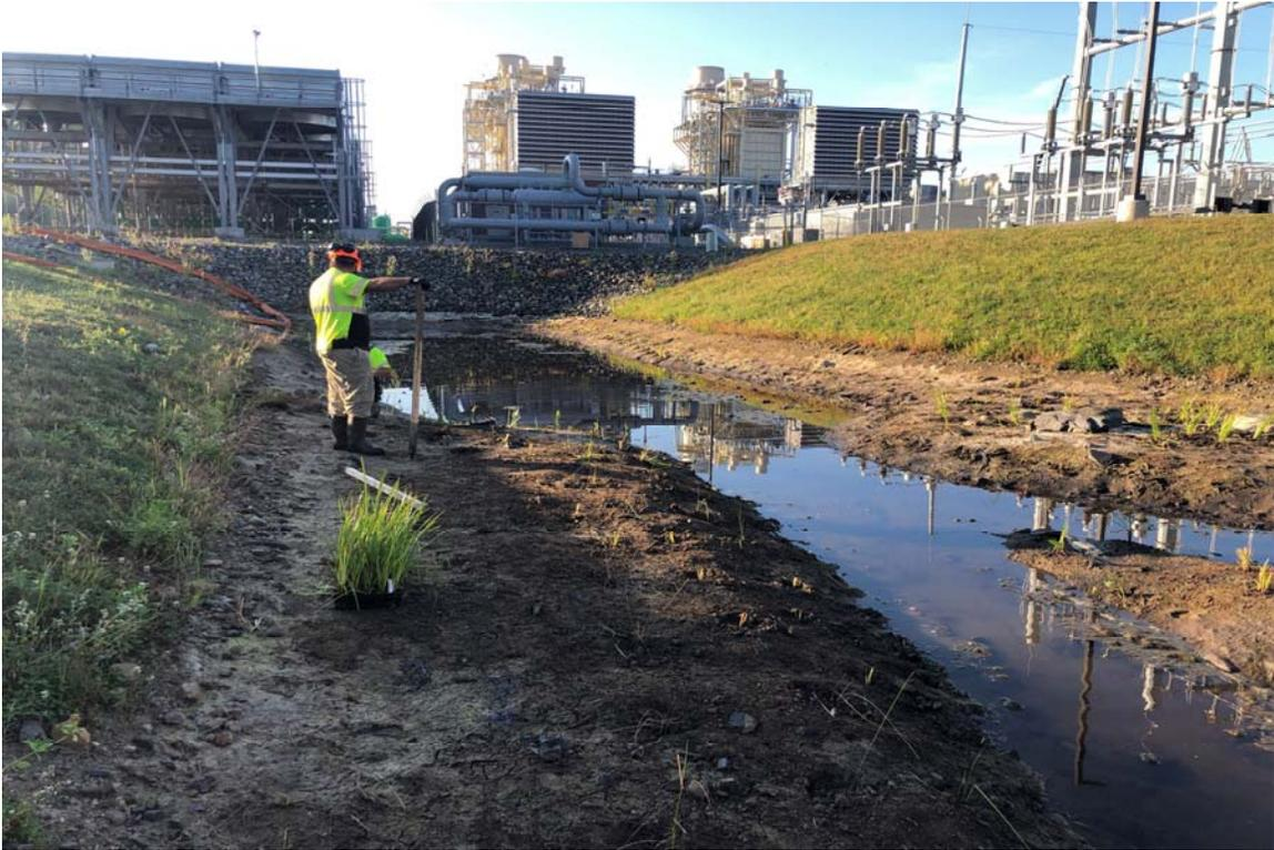
Photo 17: View of Basin 'B' high and low marsh replanting work looking south with micropool in background.
