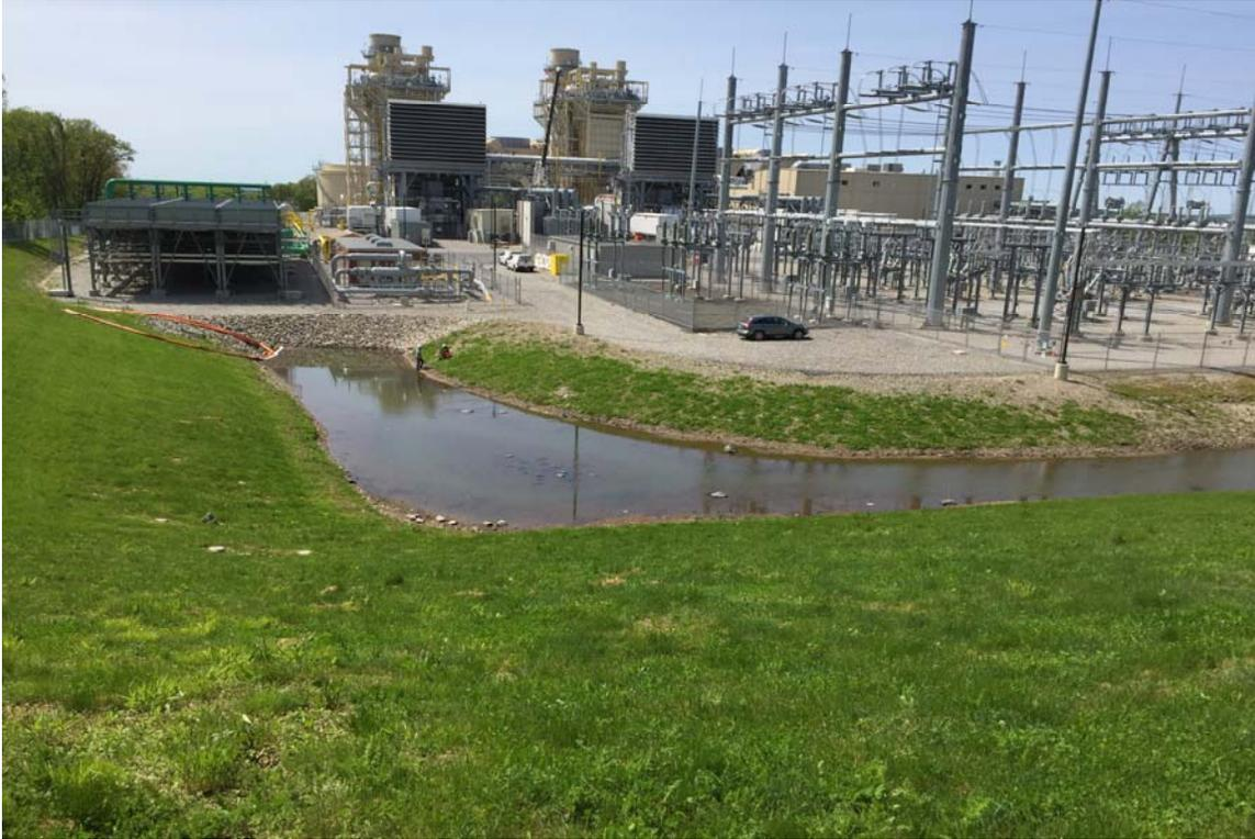
Photo 11: Overview of Basin 'B' (north basin) looking south at high and low marsh zones and micropool (in background).
