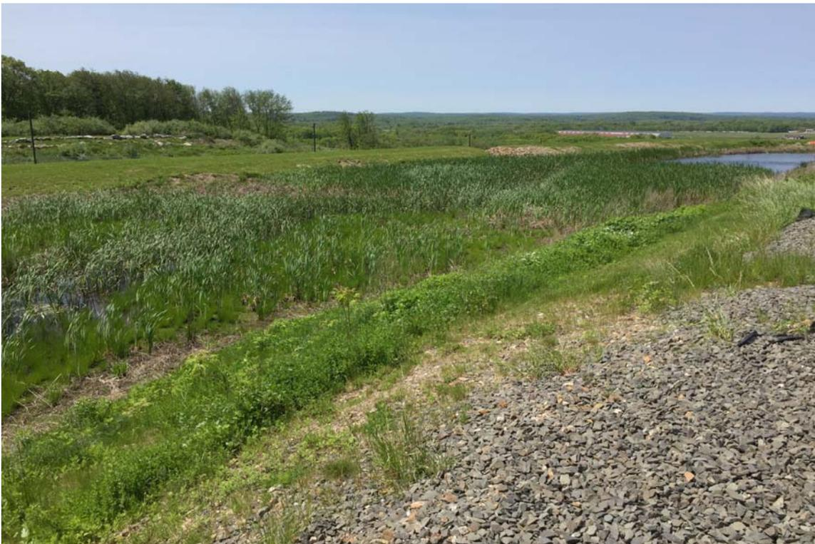
Photo 2: Overview of Basin 'A' high and low marshes with micropool in far right side of photo looking southwest.
