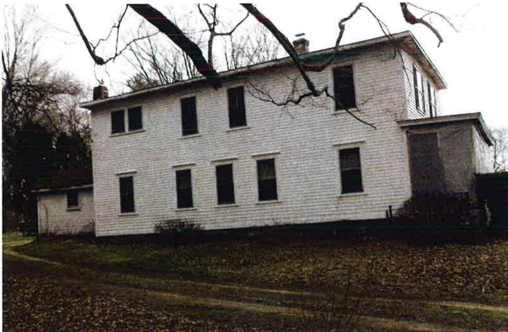
Photograph 24. Sorrow house, south façade (Photographer S.A. Reeve, March 16, 2016).
