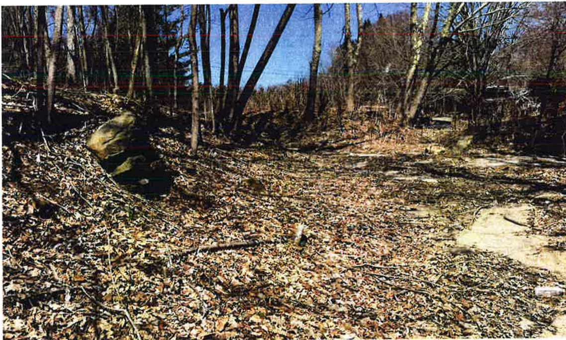
Photograph 4. Survey Area 2: graded platform and stone wall, possibly for a former outbuilding (left), drainage channel (center), and Lippitt house foundation (right). View to the west (Photographer S. Haugh, April 14, 2016).
