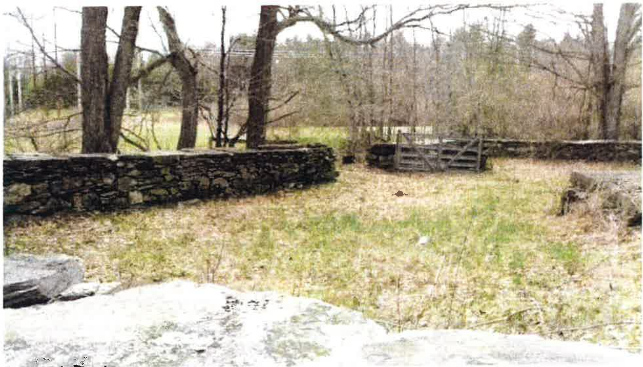
Photograph 4. Lippitt Farm Site, fieldstone walls surrounding the barnyard. View to the southwest (Photographer S.A. Reeve, March 16, 2016).
