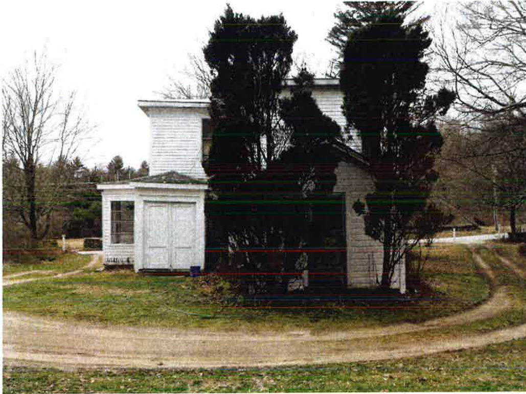
Photograph 23. Sorrow house, west façade (Photographer S.A. Reeve, March 16, 2016).
