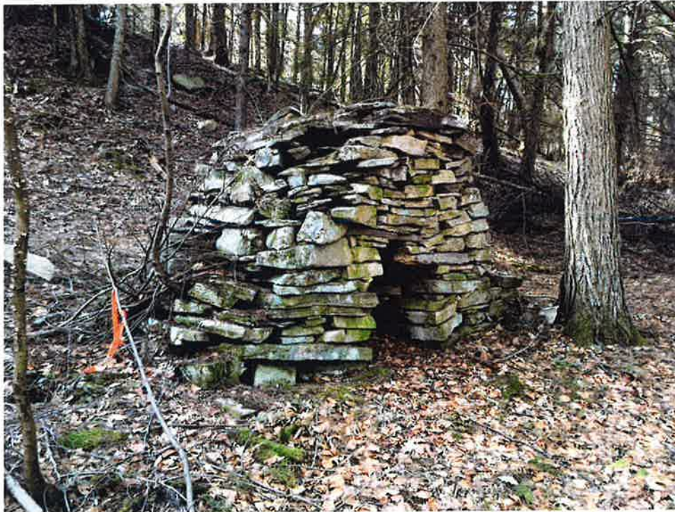
Photograph 34. Stone chimney on the Quinebaug River floodplain, west (outside) of the Project property. View to the east (Photographer S. Haugh, April 19, 2016).
