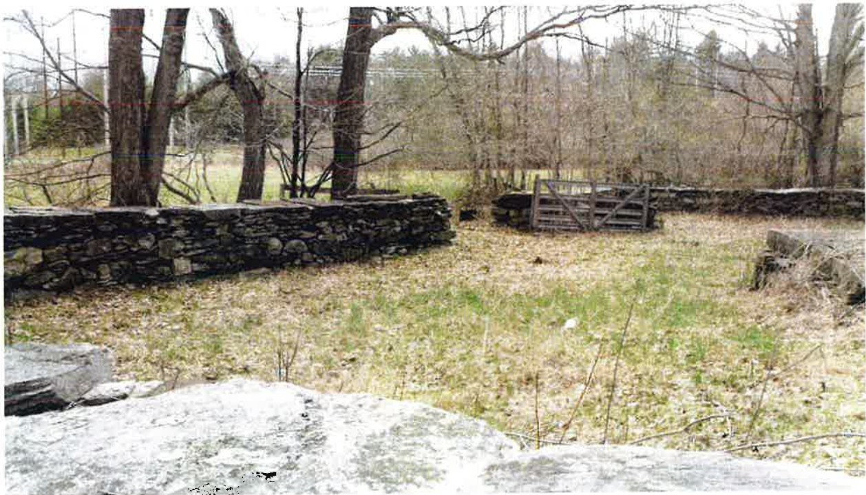
Photograph 8. Fieldstone walls surrounding the barnyard. View to the southwest (Photographer S.A. Reeve, March 16, 2016).
