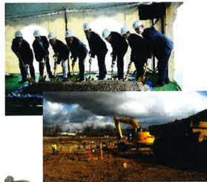
Middletown Energy Center (Ohio)
