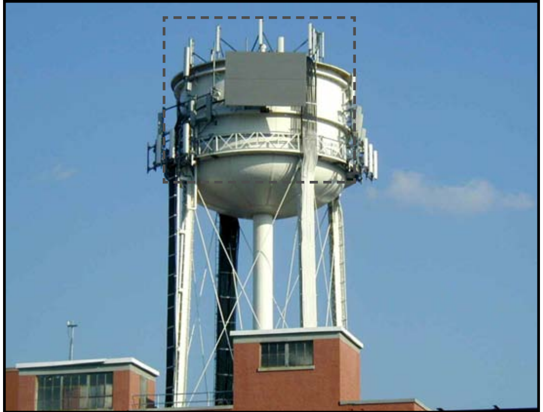
A passive microwave reflector is located at 652 Glenbrook Road in Stamford, CT. Photograph taken in December of 2006.
