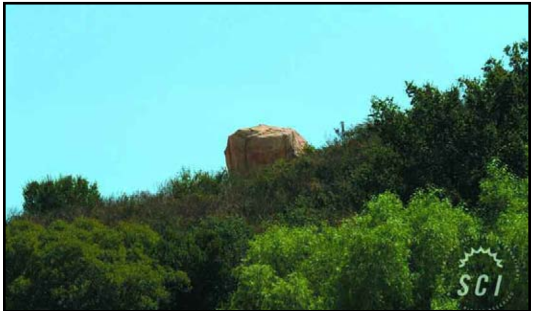
Rocky Peak Church in Chatsworth, CA. Antennas are located inside of the structure, which is made of a radio frequency transparent material. Dimensions of the structure are 11 feet 6 inches tall by 8 feet in diameter.
