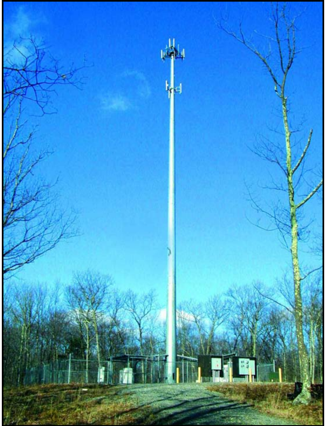
78 Route 81 in Killingworth, CT. Photograph taken in December of 2003.
