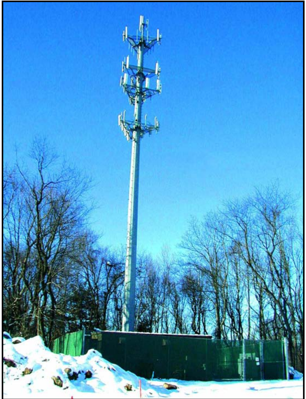
528 Wheelers Farms Road in Milford, CT. Photograph taken in January of 2004.
