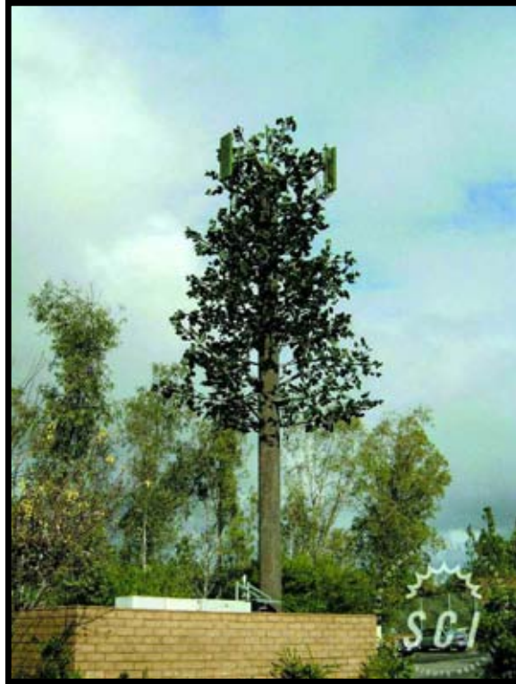
Pacifica Mormandie in Torrance, CA. The structure is 62 feet tall. Antennas are located at 55 feet agl.
