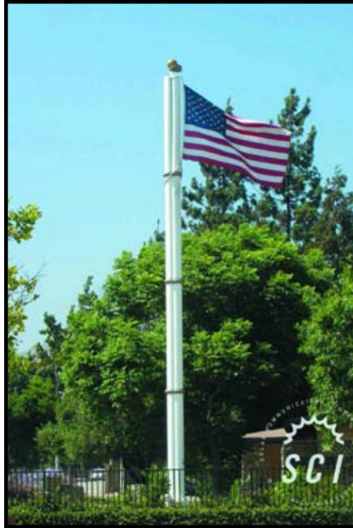
Magnolia Park in Upland, CA. The structure is 60 feet tall.
