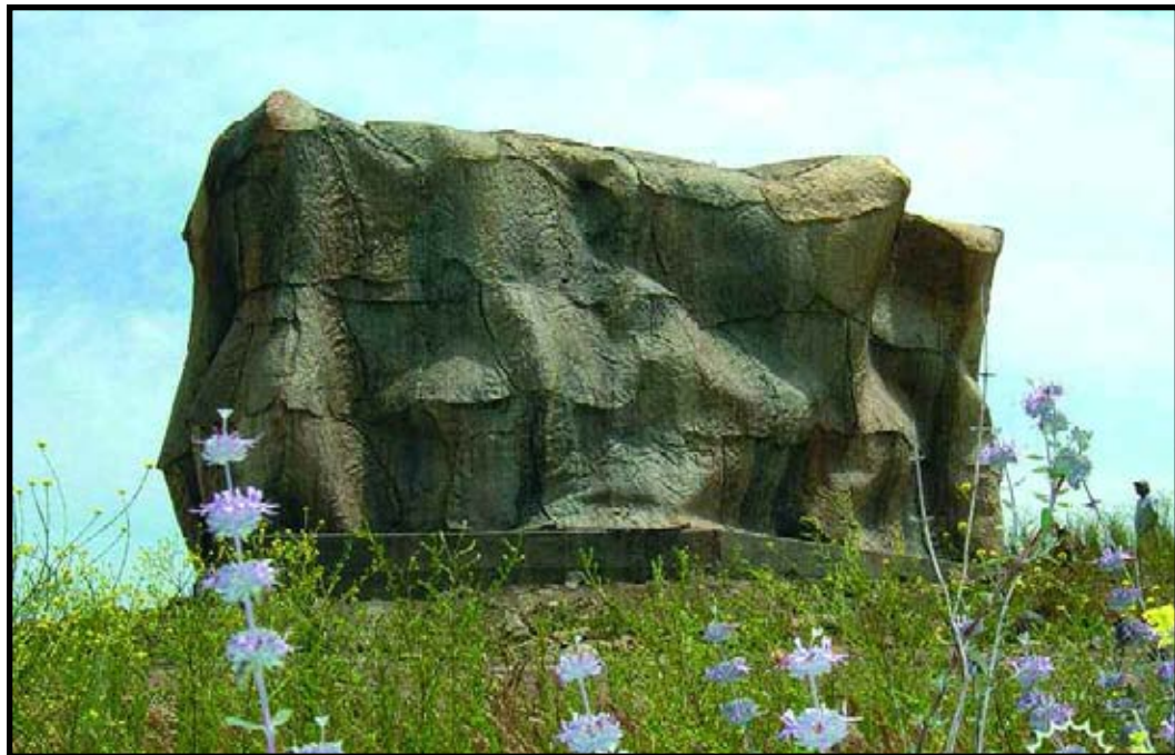
Baron Brothers' Nursery in Camarillo, CA. Antennas are located inside of the structure, which is made of a radio frequency transparent material. Dimensions of the structure are 25 feet wide by 12 feet high.
