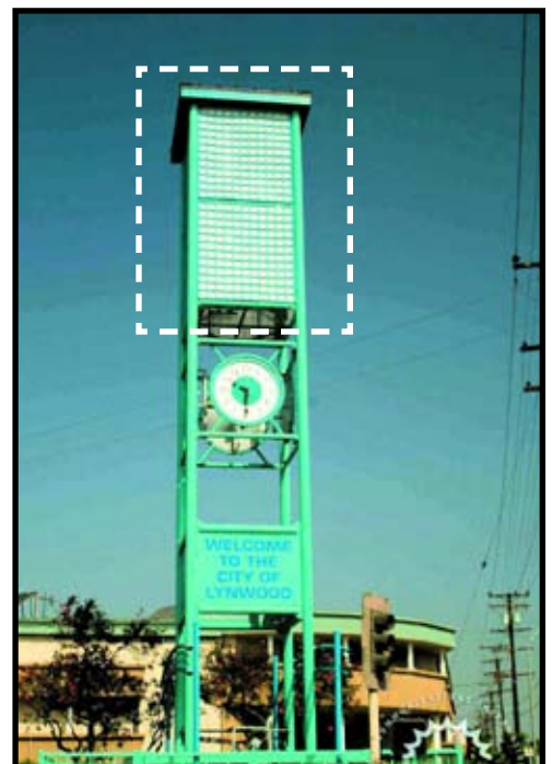
City of Lynwood, CA. Dimensions of the structure are 60 feet tall by 8 feet wide.
