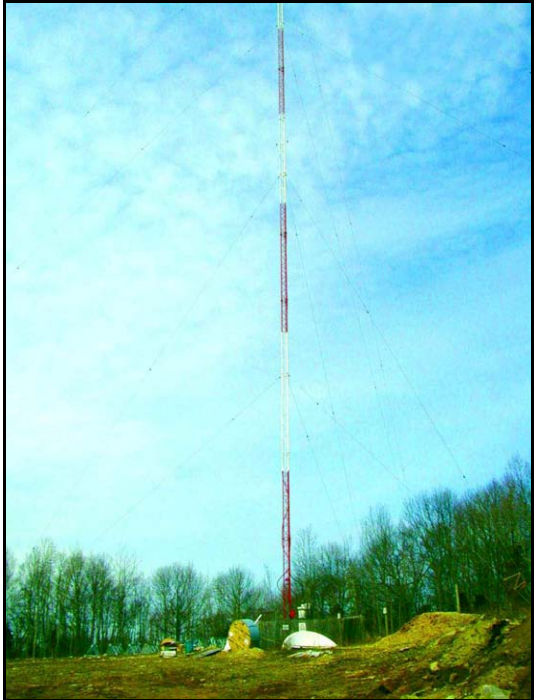
99 Briar Hill Road in Groton, CT. Photograph taken in April of 2004.
