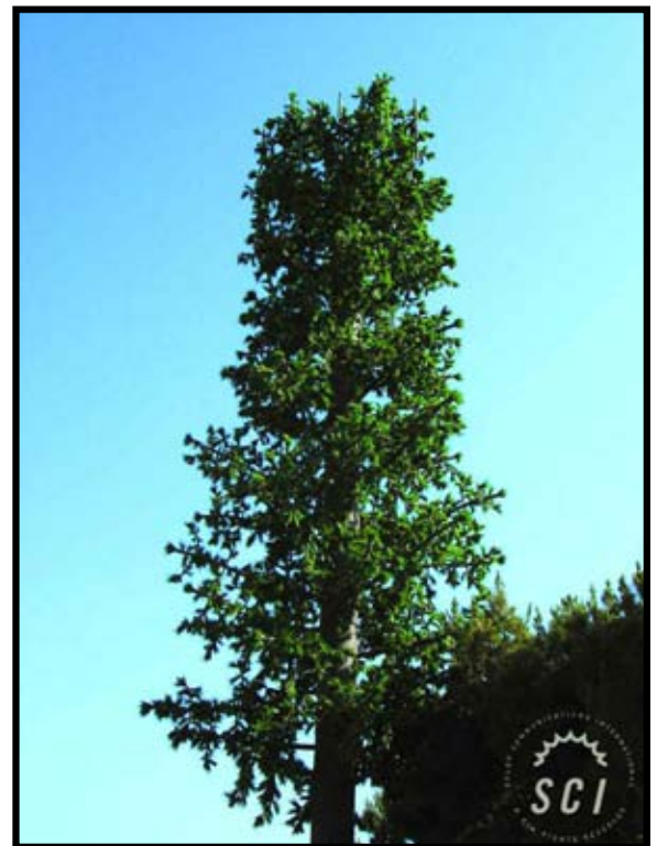
Pacifica Mormandie in Torrance, CA. The structure is 62 feet tall. Antennas are located at 55 feet agl.
