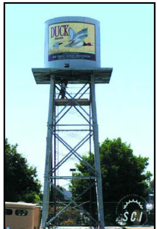
Via Verde in San Dimas, CA. The structure is 60 feet tall. Antennas are mounted within the water tank at 58 feet agl and 47 feet agl.
