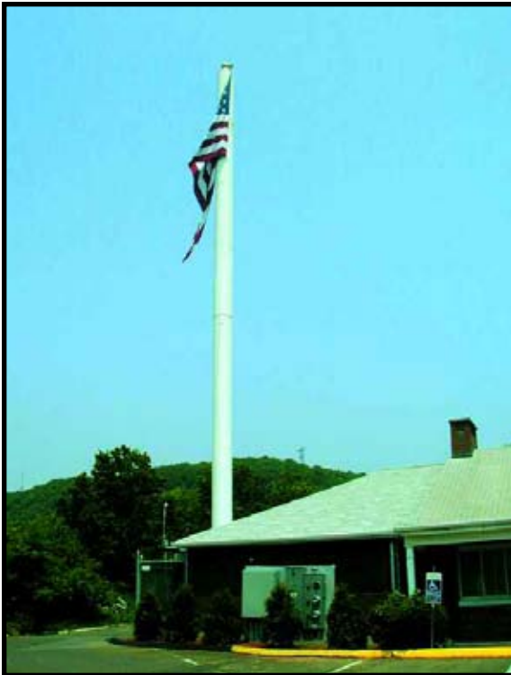
100 Pond Lily Avenue in New Haven, CT. Antennas are located within the flagpole structure and equipment is housed within a brick façade that matches the building. Photograph taken in June of 2006.
