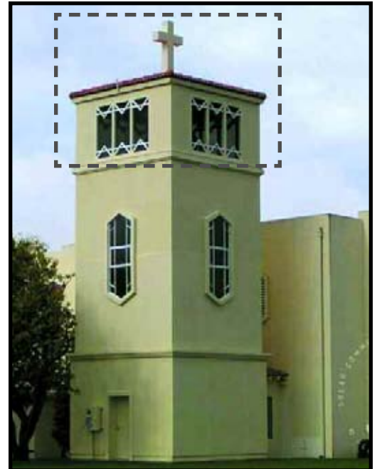
Montfort Church in Santa Maria, CA. She structure is 50 feet tall. Antennas are located at 50 feet and 42 feet agl.
