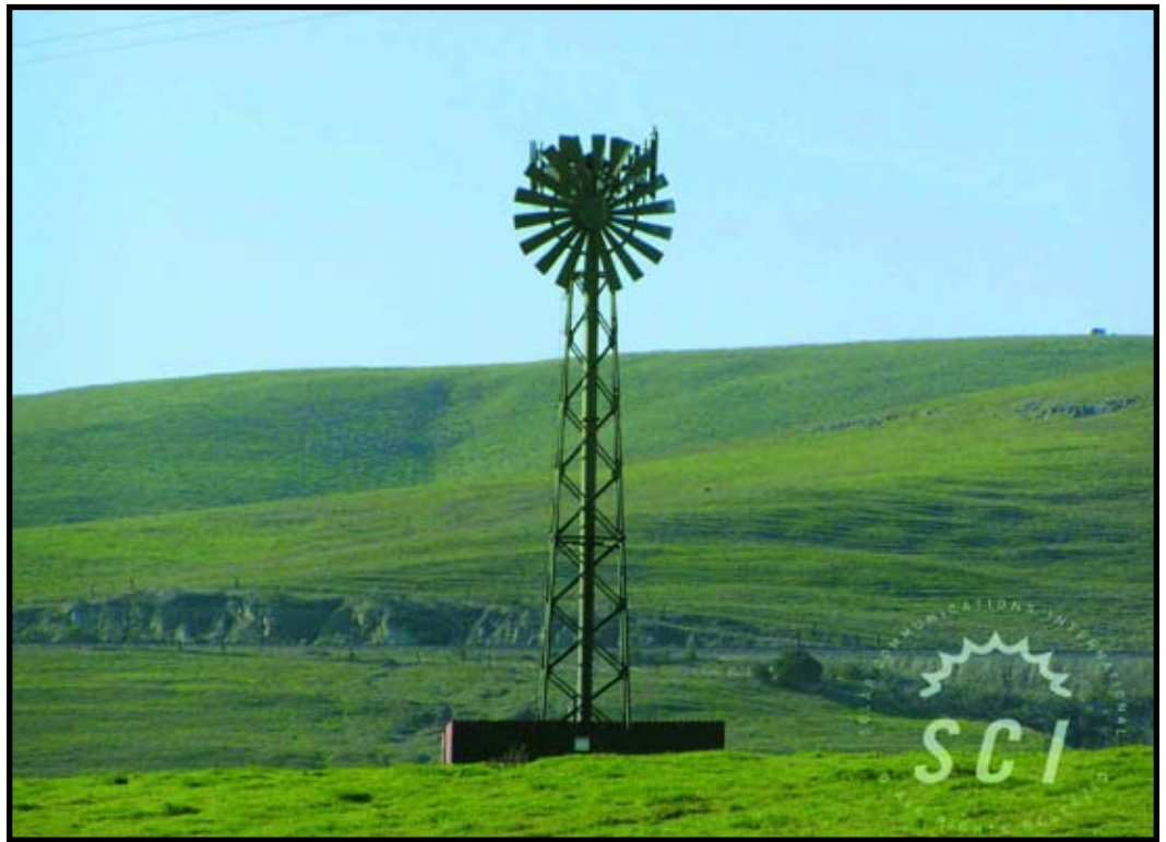
Betteravia Properties in Santa Maria, CA. The structure is 50 feet tall. Antennas are located at 48 feet agl.
