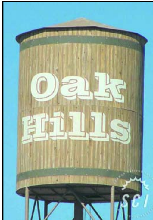
Cajon Pass in Oak Hills, CA. The structure is 90 feet tall. Antennas are within the water tank structure at 80 feet 8 inches agl and 70 feet agl.
