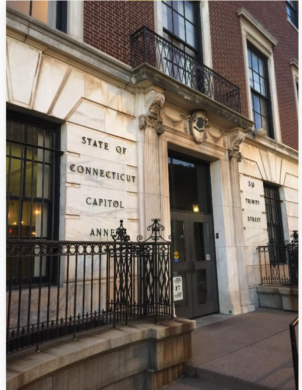
Figure 3 - Photo of State of Connecticut Capitol Annex Building, Office of Chief Public Defender. Photo contributed by: CJIS Roadmap Technical Writer, Carolyn Denesha
