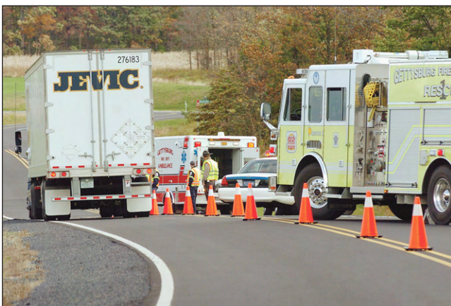
Figure 4.1—A TTC zone is established by responders to a roadway incident.
