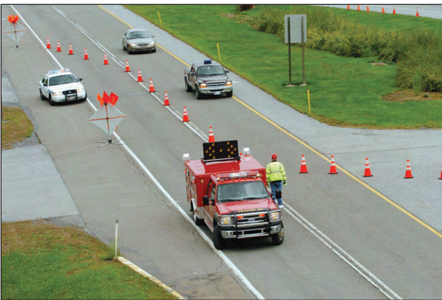
Figure 4.11—Flaggers should be in the lane adjacent to the moving traffic.
