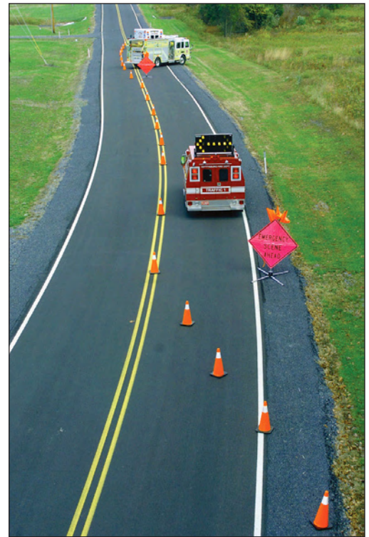
Figure 4.10—The initial stages of establishing a TIMA.
