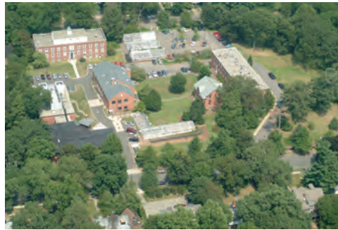
Main Laboratories, New Haven
