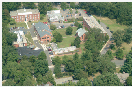
Main Laboratories, New Haven
