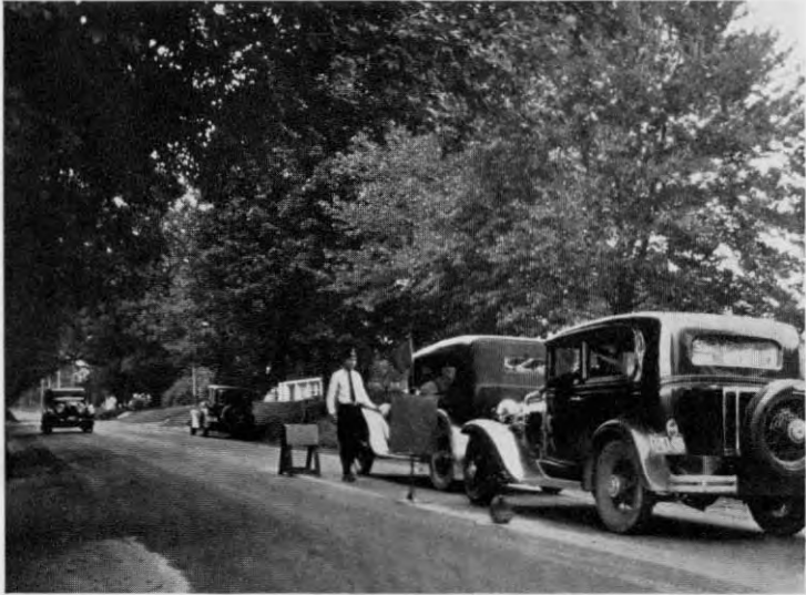
a. View of road patrol inspection at the Easton-Bethel town line on the Bridgeport-Danbury highway.
