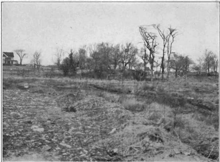
b. Same area after ditching and filling part of the foreground.
