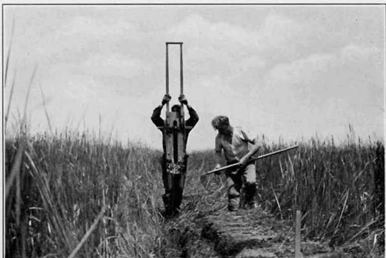
a. Ditching through cat-tails. Quinnipiac marsh, Hamden. Spade raised to cut sod.
