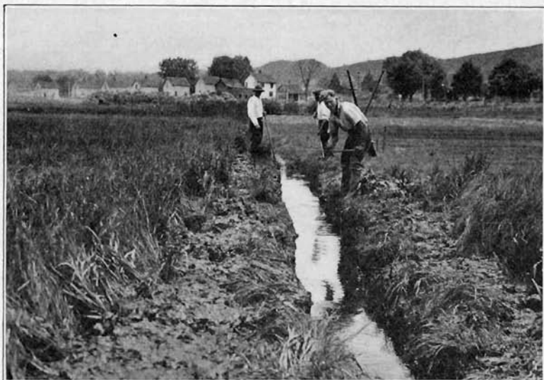
a. View in Quinnipiac marsh, showing workmen cleaning old ditch.
