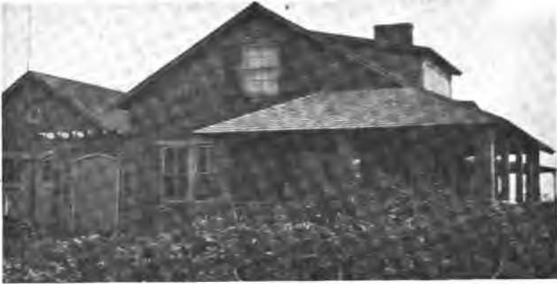
a. General View of Invaded House.
